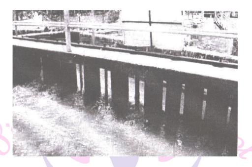
iii) The water is then allowed to settle in a large tank sloped towards the middle. Solids like faeces settle at the bottom and are removed with a scraper.
